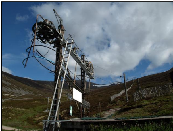
Ski infrastructure in the Cairngorms NP
