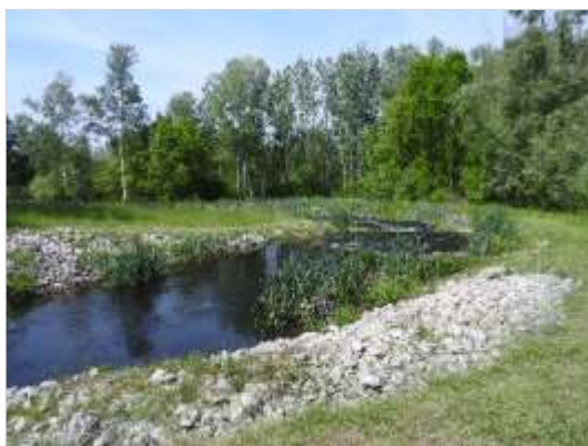
Picture 18. On the left: fish ladders, on the right: water level controlling system-construction.
