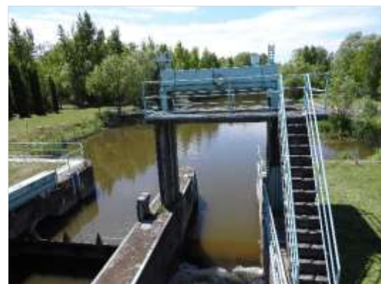
Picture 18. On the left: fish ladders, on the right: water level controlling system-construction.
