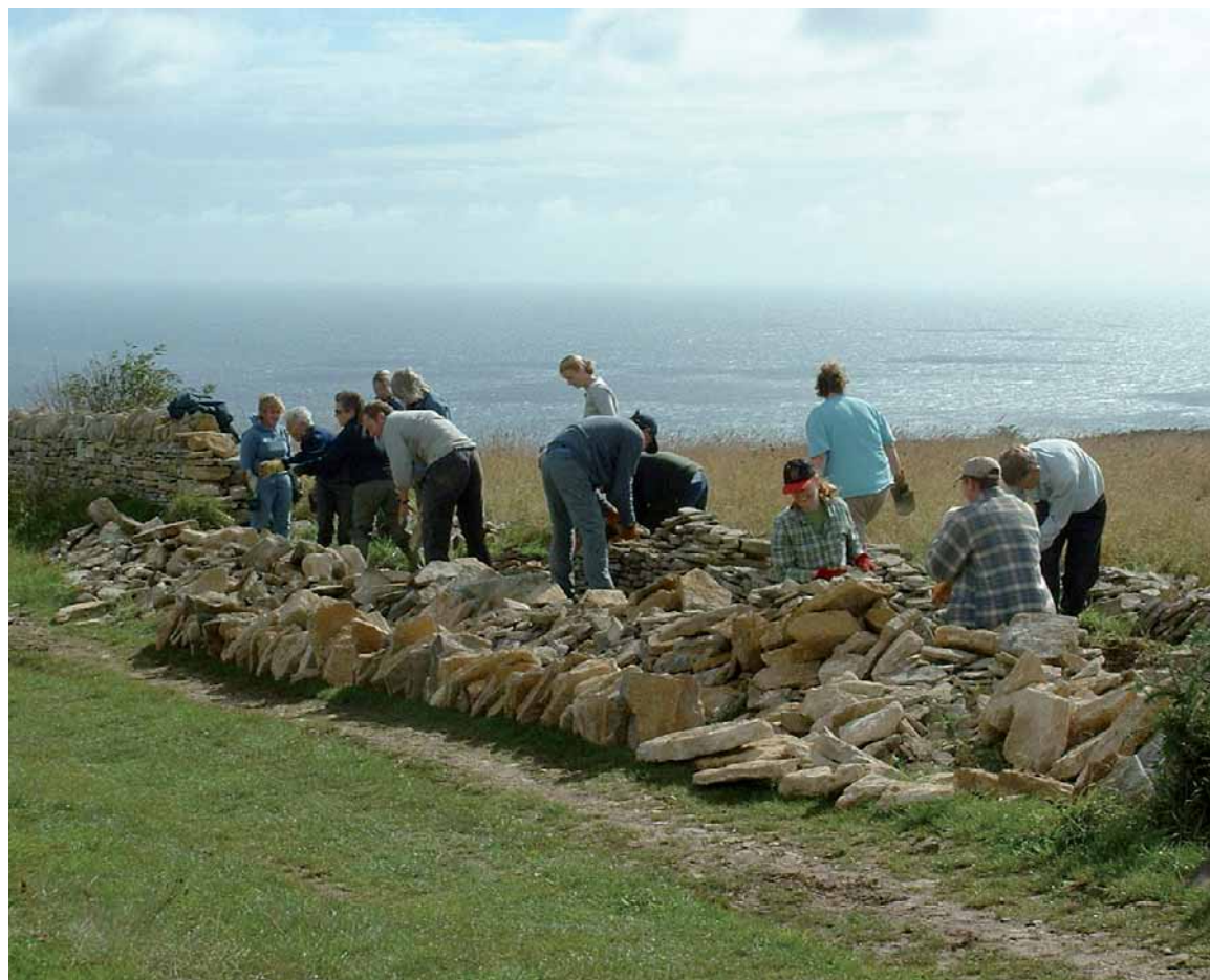
Volunteers preparing to rebuild a section of drystone wall in South Devon AONB. Picture: BTCV
