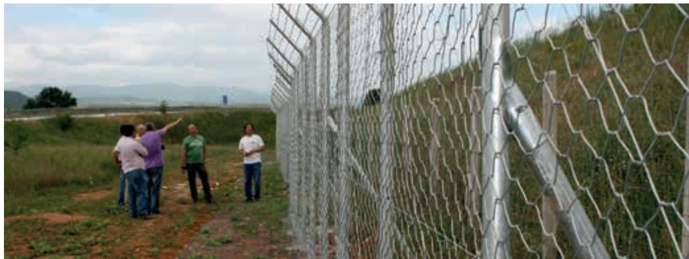
Fig. 9. Installing the “bear-proof” reinforced fence on the highway after successful efforts of CALLISTO.
