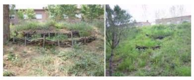
Sinking of wooden stakes where the material is structured horizontally.
