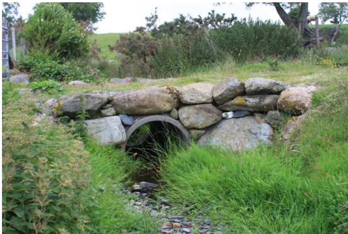
Photo 18 - Small bridge to avoid banks' erosion by the cattle. Snowdonia NP (July 2010, U. Biereżnoj)
