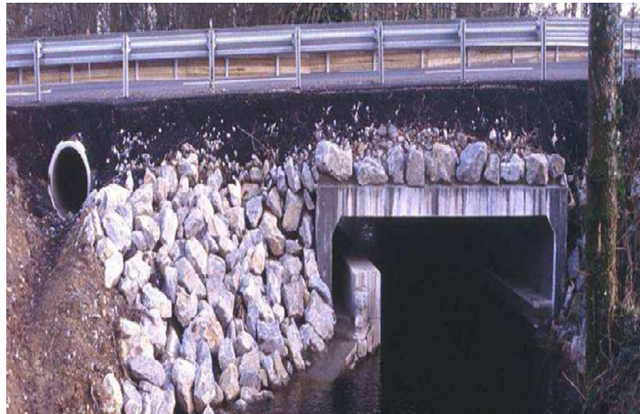
Photo 9 - Tunnel under the road bridge built for otters, Briere RNP (M. Marquet)
