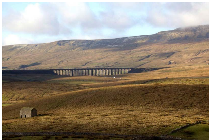
The magnificent 19th railway viaduct looks remote but has become a major visitor honeypot (photo: Hilary Fenten)
