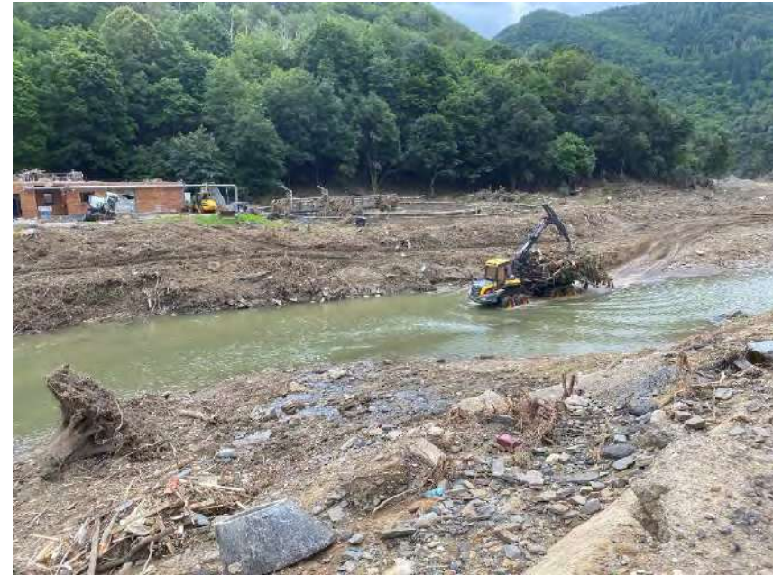
Wastewater treatment plant Altenahr
